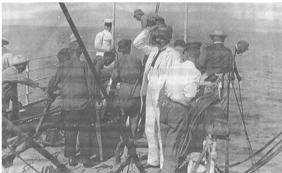
Kabel-reparation i Manila-
